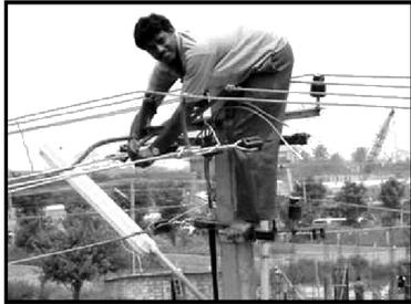
**FIGURE 8: Illegal connection of electricity**
