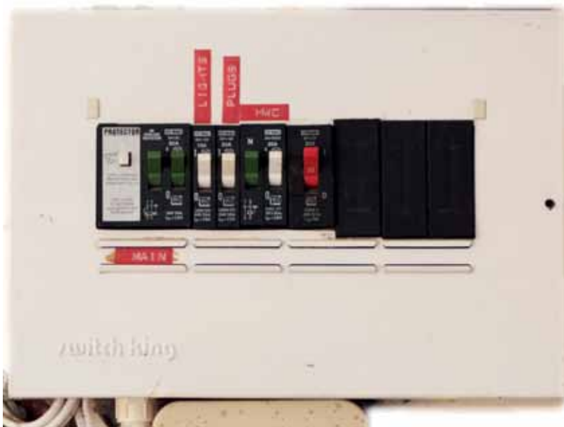
Figure 2: An electrical distribution board with circuit breakers
